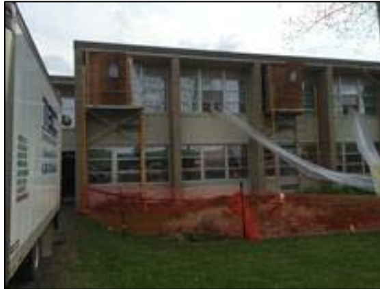
Classroom Abatement – Code-Compliant Barriers and Negative Air in Place
