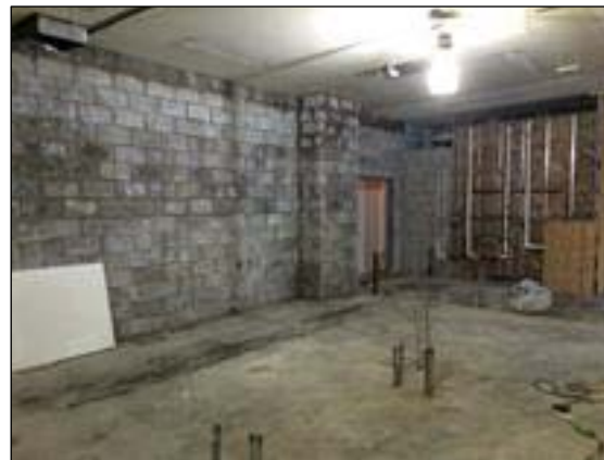
Masonry and Metal Stud Wall Construction
