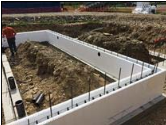
Insulated Concrete Forms being Erected
