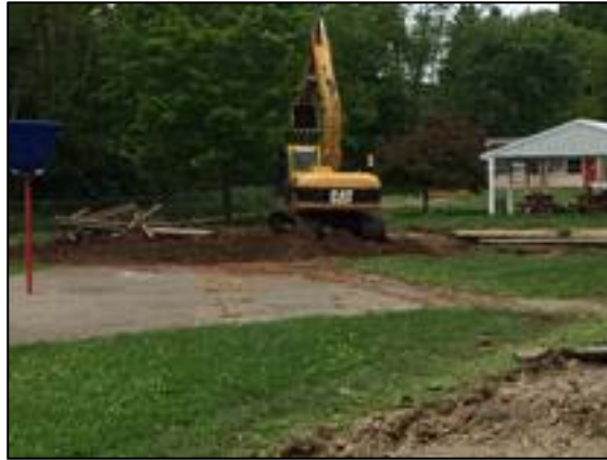
Removing Existing Walkways
