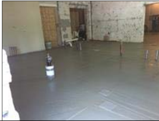
Pouring Concrete Floor in Kitchen
