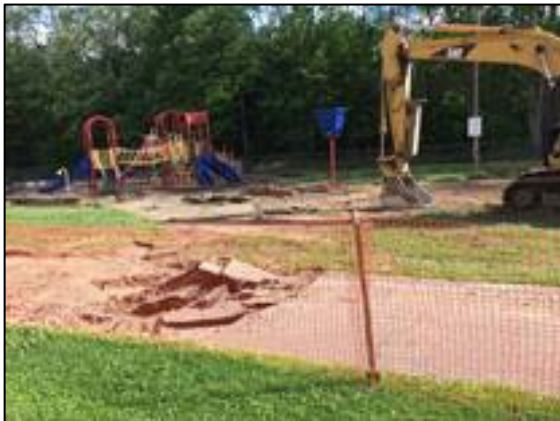
Removing Existing Walkways
